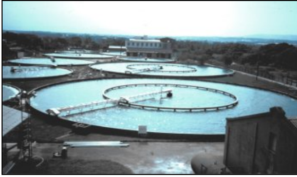
Figure 2.1.3: Circular ponds ( Chlorella production in Taiwan). 17
